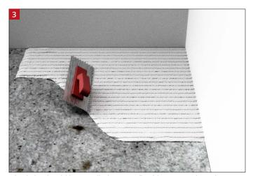
Ultralight should be installed using a flexible, cement-based adhesive. The adhesive should be trowelled out and combed through using a 6 mm x 6 mm ( $\frac{1}{4}$ " x  $\frac{1}{4}$ ") square notch trowel to give a ribbed bed, any slight depressions in the subfloor being filled by the mortar.
